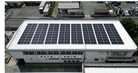
After introduction of solar power generation facilities
