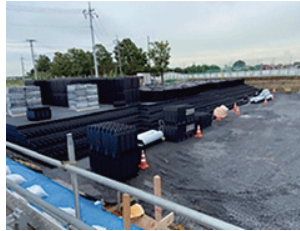
Construction of the storm water detention tank
