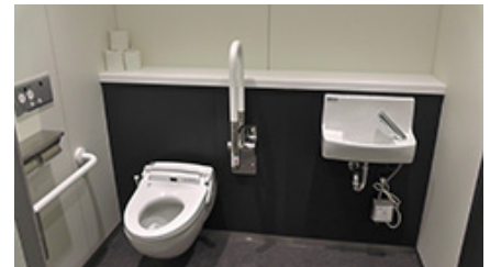
Toilet that can be easily used by people in wheelchairs at the new West Main Building at the Gunma Manufacturing Division
